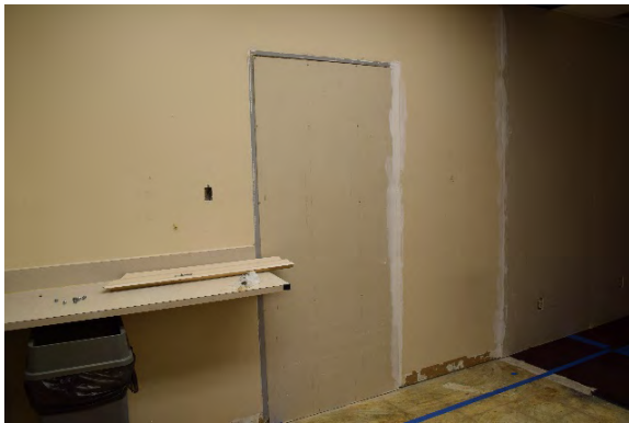
Picture 1 Office Renovation
